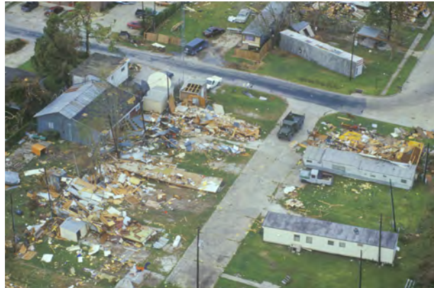
Damage from Hurricane Andrew. By: spiritofamerica/stock.adobe.com
